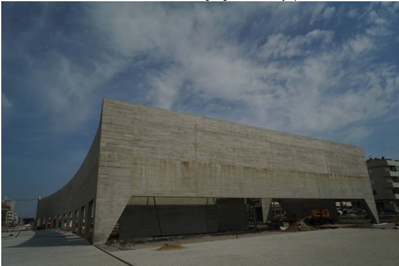
Rehabilitation of the ongoing Canal Railway Space
